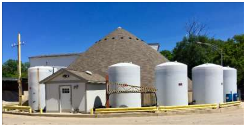
Figure 4: Salt dome, liquid storage tanks and pump control facility.
