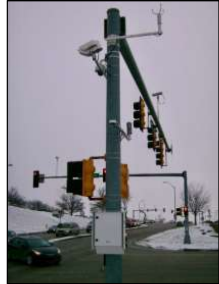
Figure 7: Typical RWIS equipment.
