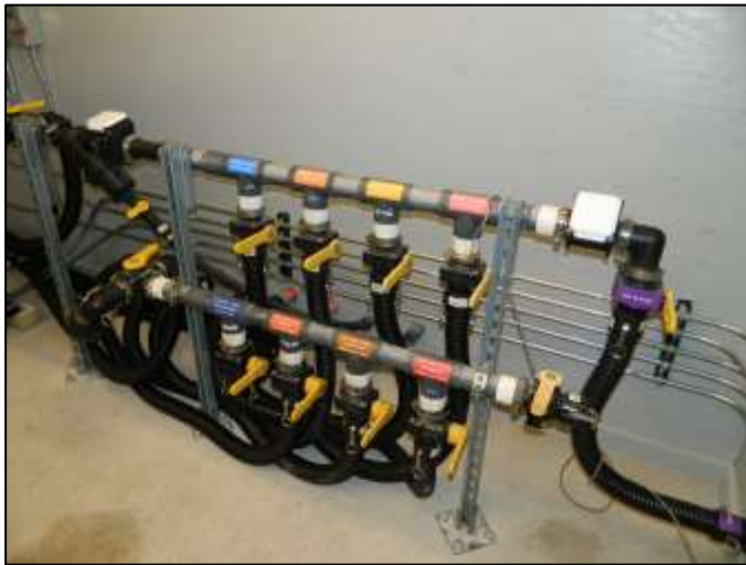
Figure 3: Liquid distribution and recirculation controls.
